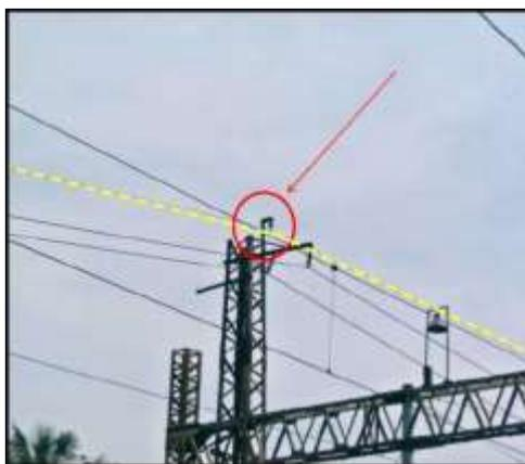
**Figure14.** Ground wire/OHGW ungrounded.
