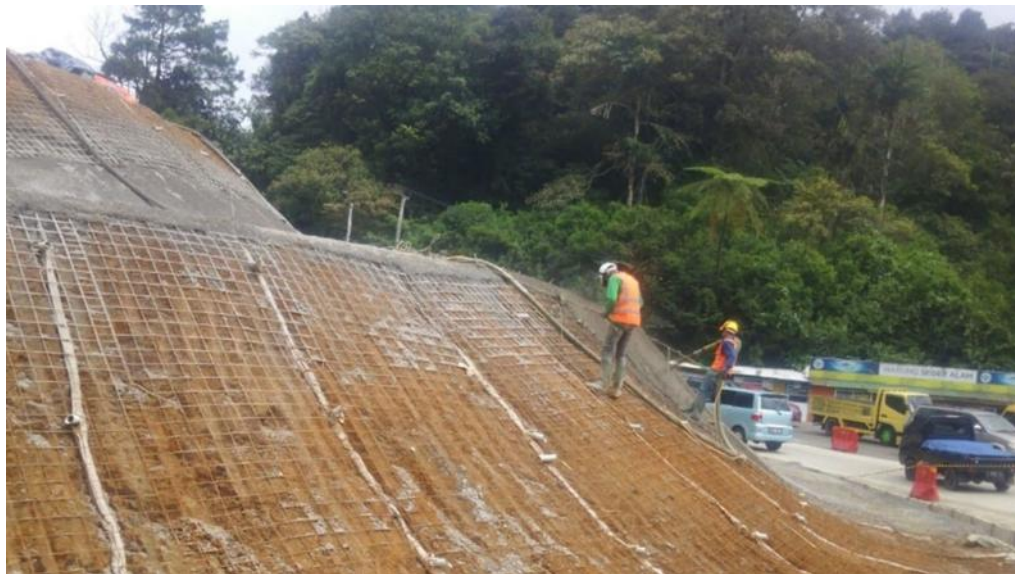
Gambar 2. Soil Nailing: Teknik Modern Stabilisasi Tanah
